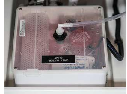
GRAY WATER SUMP
