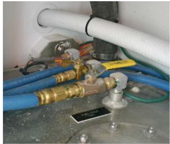
PORT TANK showing fuel shut-off for port engine and generator (center hose).
