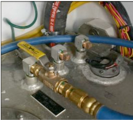
STARBOARD TANK showing fuel shut-off and top of fuel level sensor (right center)
