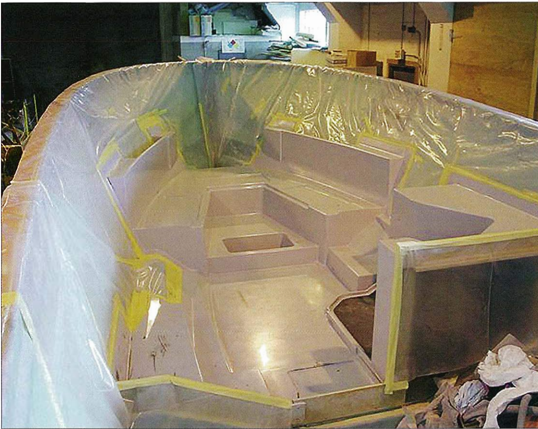
The 34z's FRP pan is outsourced to Meikle Marine & Machine in Tiverton, Rhode Island, and trucked to Boston BoatWorks.
